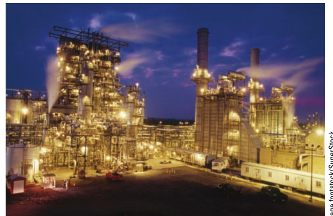
Figure 15-4 Science: When crude oil is refined, many of its components are removed at various levels, depending on their boiling points, of a giant distillation column (left) that can be as tall as a nine-story building. The most volatile components with the lowest boiling points are removed at the top of the column. The photo above shows an oil refinery in the U.S. state of Texas.
