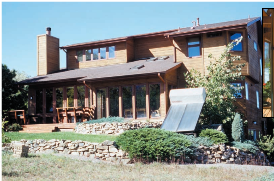
Figure 16-12 This passive solar home (left) in Golden, Colorado (USA), collects and stores incoming solar energy which provides much of its heat in a climate with cold winters. Such homes also have the best available insulation in their walls and ceilings, and energy-efficient windows to slow the loss of stored solar energy. Notice the solar hot water heating panels in the yard. Some passive solar houses like this one (see photo on right) in Dublin, New Hampshire (USA), have attached sunrooms that collect incoming solar energy.
