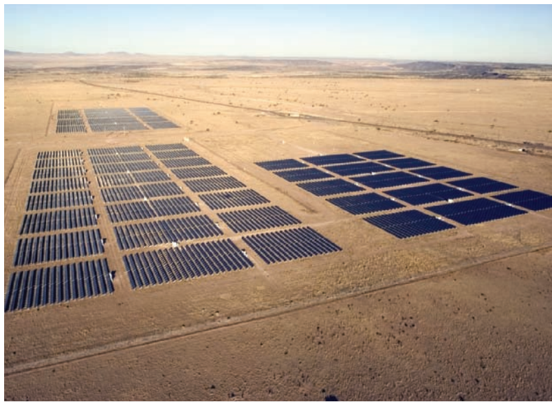
Figure 16-20 This solar-cell power plant in the U.S. state of Arizona near the city of Springerville has been in operation since 2000 and is the world's largest solar-cell power plant. Analysis shows that the plant, which is connected to the area's electrical grid, paid back the energy needed to build it in less than 3 years.
