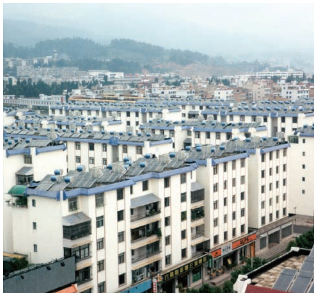
Figure 16-13 Rooftop solar hot water heaters, such as those shown here on apartment buildings in the Chinese city of Kunming in the province of Yunnan, are now required on all new buildings in China, and their use is growing rapidly in urban and rural areas.
