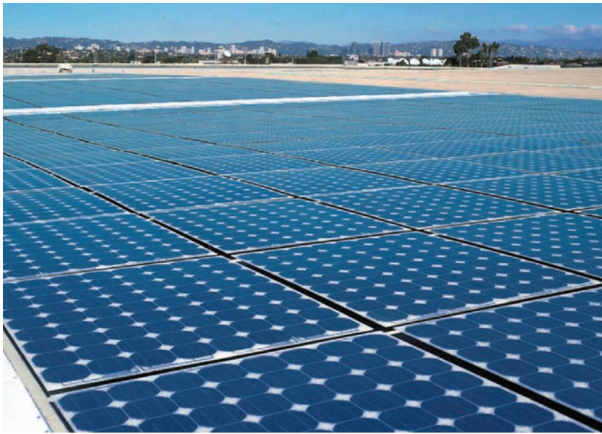
Figure 16-18 Solutions: Photovoltaic (PV) or solar cells can provide electricity for a house or building using conventional solar panels such as those shown here (left) on the roof of a U.S. Postal Service processing and distribution center in Inglewood, California. They can also be incorporated into metal roofing materials that can simulate the look of ceramic roof tiles, as well as slate, wooden shake, or asphalt shingles in a wide variety of colors. A new plug-and-play light-weight modular rooftop solar cell system can be snapped together and installed in a few hours. In addition, new, flexible, thin-film solar cells (right) or even more efficient tiny silicon nanorods (made with the use of nanotechnology) can be applied to roofs, windows, building walls, bridges—almost any surface, even T-shirts.
