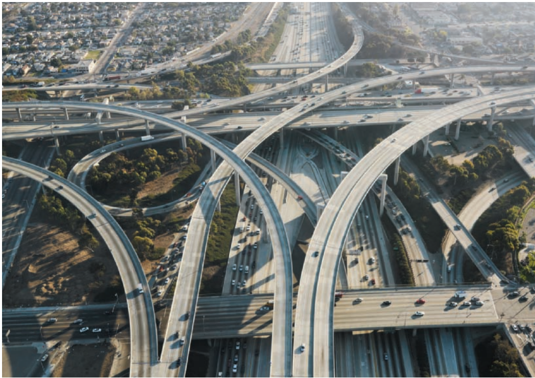
Figure 22-13 Concrete cloverleaves like this tangled network of thruways in the U.S. city of Los Angeles, California, are found in most of the world's increasingly car-dependent cities.
