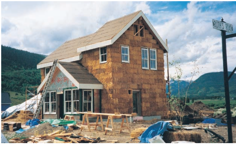
Photo 8 Energy efficient straw bale house in Crested Butte, Colorado (USA) during construction.
