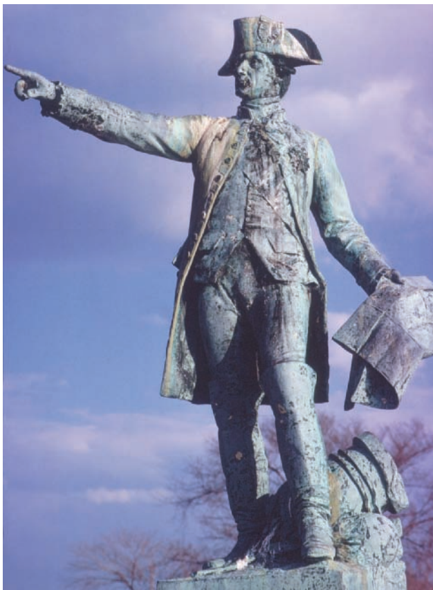
Figure 18-7 Acid deposition and other forms of air pollution have corroded this statue in Newport, Rhode Island (USA).
