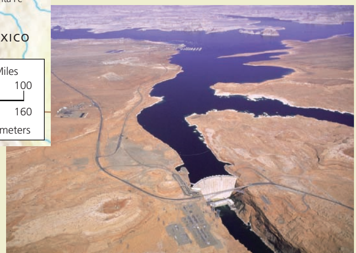
Figure 13-2 The Glen Canyon Dam across the Colorado River was completed in 1963. Lake Powell behind the dam is the second largest reservoir in the United States.
