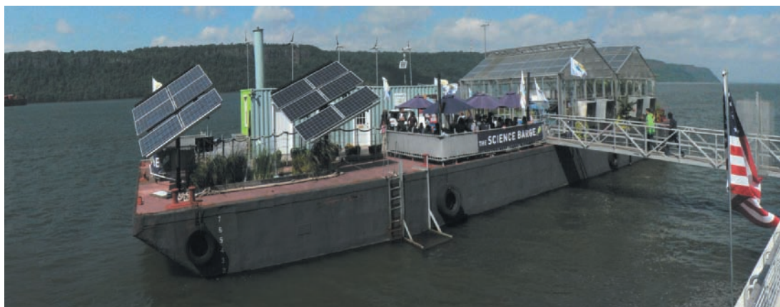
Figure 12-36 The Science Barge located in Yonkers, New York is a prototype for a sustainable urban farm. It uses a water purification and recirculating system and renewable energy to raise vegetables hydroponically (Figure 12-6) with no use of pesticides, no runoff of polluted water, and no net emissions of carbon dioxide.
