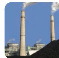
Coal-fired power plant emissions
