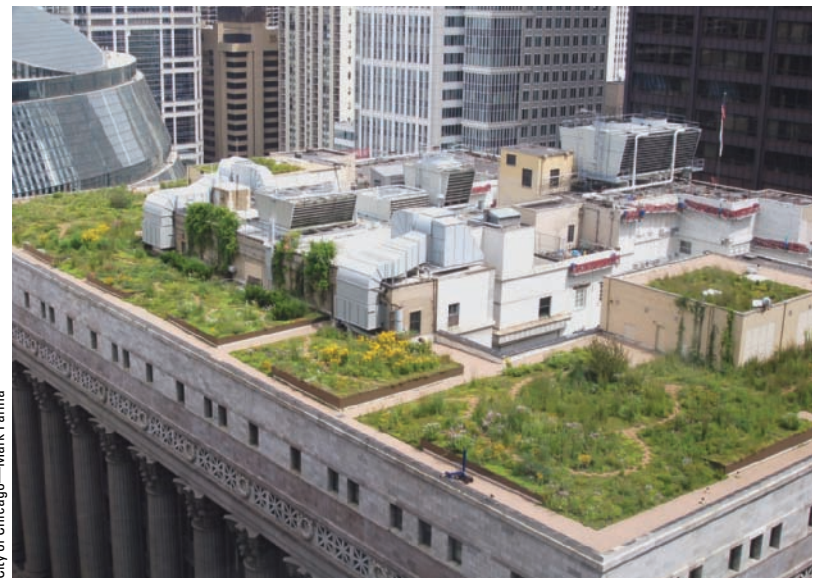
Figure 16-8 City Hall in Chicago, Illinois (USA), has a green or living roof —an important part of the city's efforts to become a more sustainable green city. Such a roof can save energy used to heat and cool the building. It absorbs heat from the summer sun, which would otherwise go into the building, and it helps to insulate the structure and retain heat in the winter. In addition, it absorbs precipitation, which would normally become part of the city's storm water runoff and add to pollution of its waterways.
